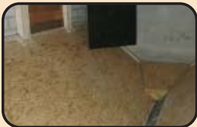
Pelletchamber with angled floor and auger collector
